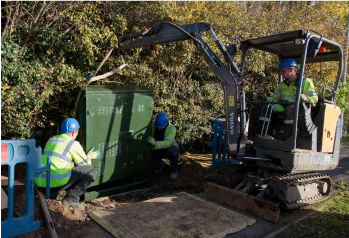
**Figure:** Installation of a fibre street cabinet in the rural village of Spaldwick
