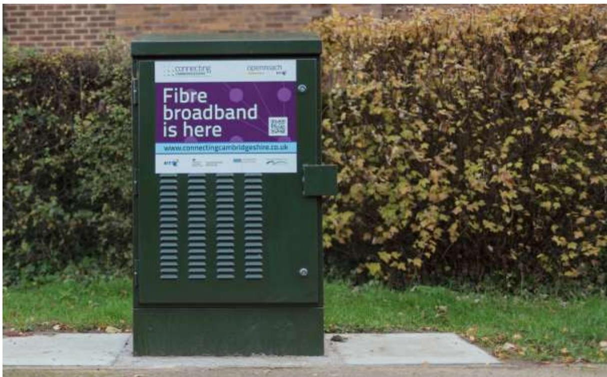
**Figure:** New fibre broadband street cabinet used to deliver fibre broadband to homes and businesses in Cambridgeshire
